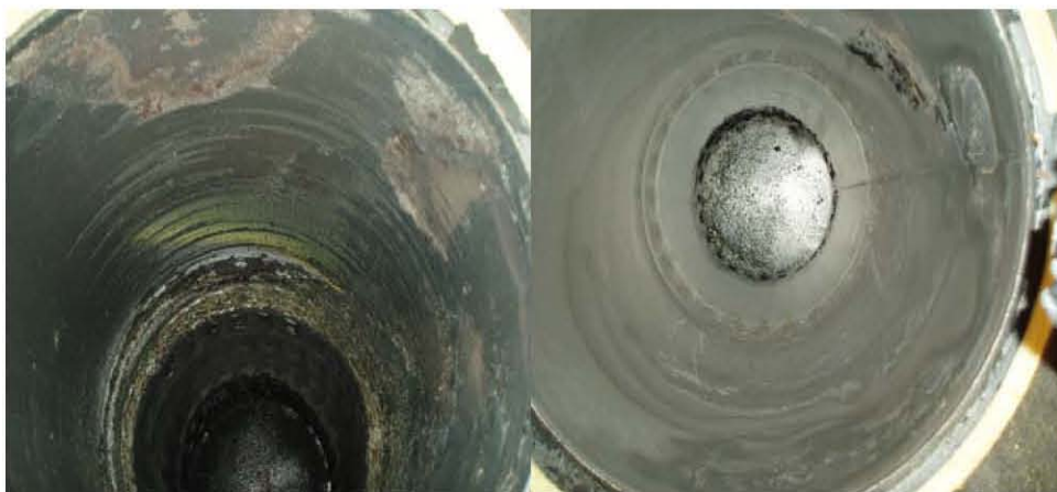
Figure 24 Condensing boiler before and after cleaning by water wash
