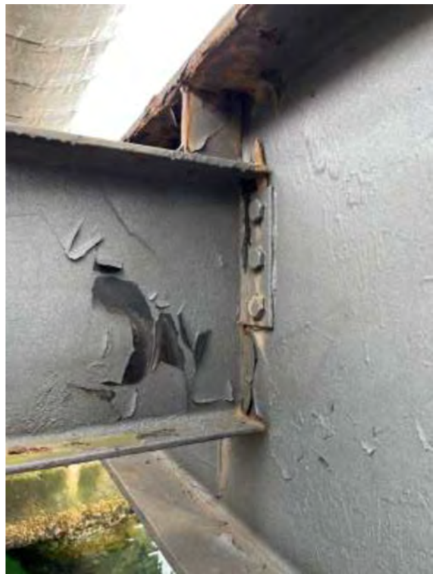
Photo 4 - North Girder at Span A and typical bolted beam to girder connection.
