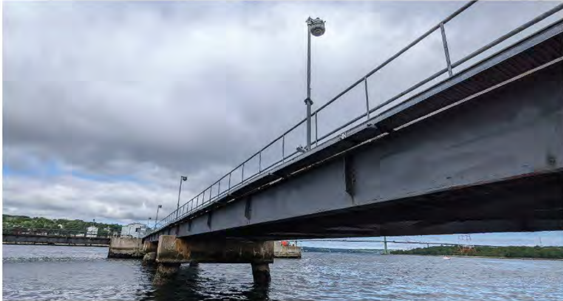
Photo 5: General photo showing the exterior of Girder 1 as identified in the Inspection Layout Sketch found in Appendix A. The coatings appear to be in good condition, with some local breakdown around the corners of the flange, and some local blistering on the webs. Local corrosion observed in various locations along the girder.
