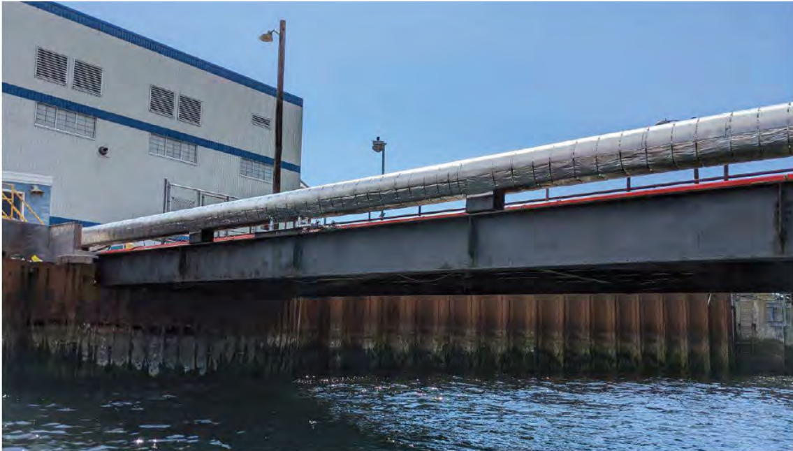
Photo 10: General photo showing the exterior of Girder 4 as identified in the Inspection Layout Sketch found in Appendix A. The coatings appear to be in good condition, with some local breakdown around the corners of the flange, and some local breakdown on the webs, flanges, and stiffeners. Local corrosion observed in various locations along the girder.
