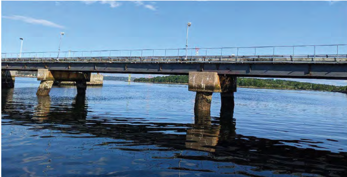
Photo 1: General photo of the configuration of the wharf structure showing the South primary girders and piers 1 and 2.
