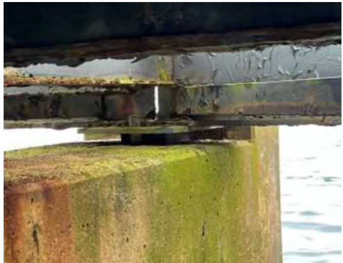
Photo 29 - Bearing plate and anchorage to pile caps observed to be in fair condition.
