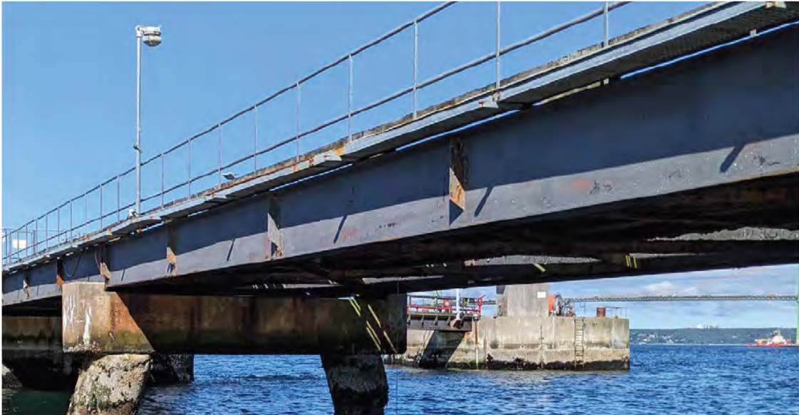
Photo 6: General photo showing the exterior of Girder 2 as identified in the Inspection Layout Sketch found in Appendix A. The coatings appear to be in good condition, with some local breakdown around the corners of the flange, and some local blistering on the webs. Local corrosion observed in various locations along the girder.
