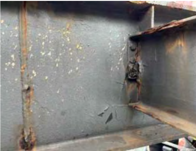
Photo 32 - South side of North Girder
