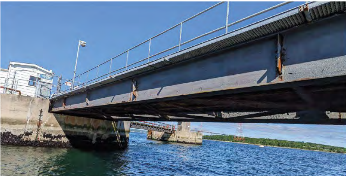
Photo 7: General photo showing the exterior of Girder 3 as identified in the Inspection Layout Sketch found in Appendix A. The coatings appear to be in good condition, with some local breakdown around the corners of the flange, and some local flaking on the webs and stiffeners. Local corrosion observed in various locations along the girder.
