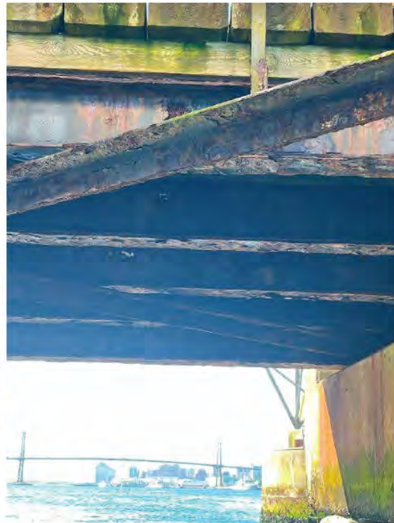
(b) Stringer 38 and Stringer 39
