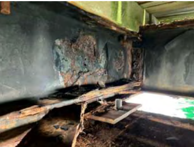
Photo 28 - Bearing plate and anchorage to pile caps observed to be in fair condition.
