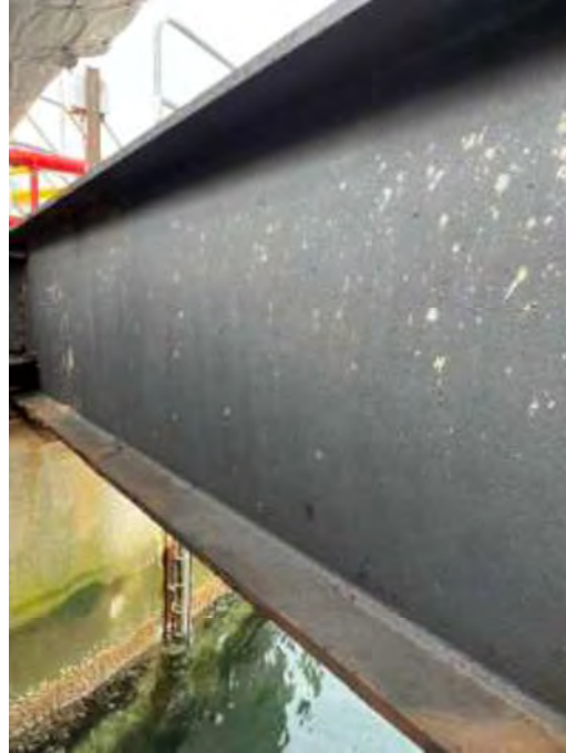
Photo 18 - North Girder (South side) at Span C in fair condition.
