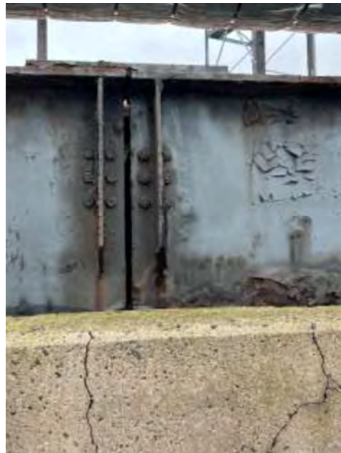
Photo 33 - Girders connection at pile caps.
