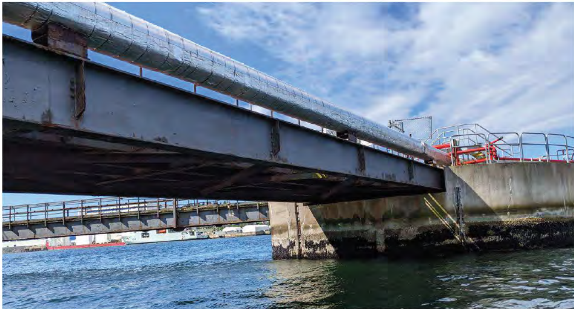
Photo 8: General photo showing the exterior of Girder 6 as identified in the Inspection Layout Sketch found in Appendix A. The coatings appear to be in good condition, with some local breakdown around the corners of the flange, and some local breakdown on the webs, flanges, and stiffeners. Local corrosion observed in various locations along the girder.
