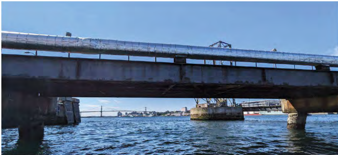
Photo 9: General photo showing the exterior of Girder 5 as identified in the Inspection Layout Sketch found in Appendix A. The coatings appear to be in good condition, with some local breakdown around the corners of the flange, and some local breakdown on the webs, flanges, and stiffeners. Local corrosion observed in various locations along the girder.
