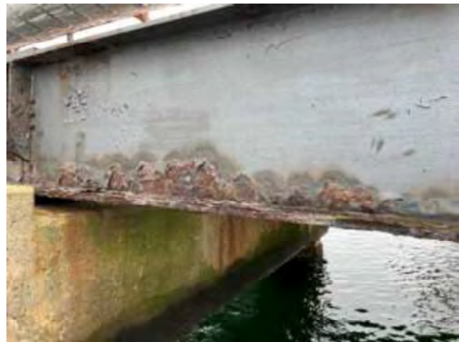
Photo 16 - South Girder at Span B in fair condition.
