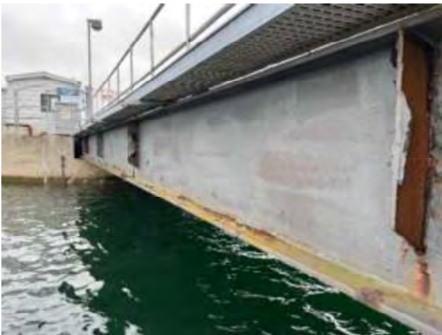
Photo 15 - South Girder at Span C in fair condition.
