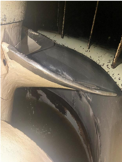
Photo 6: Turbine runner cladding and blades
