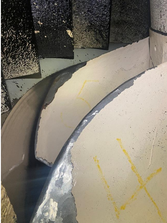
Photo 7: Turbine runner blades
