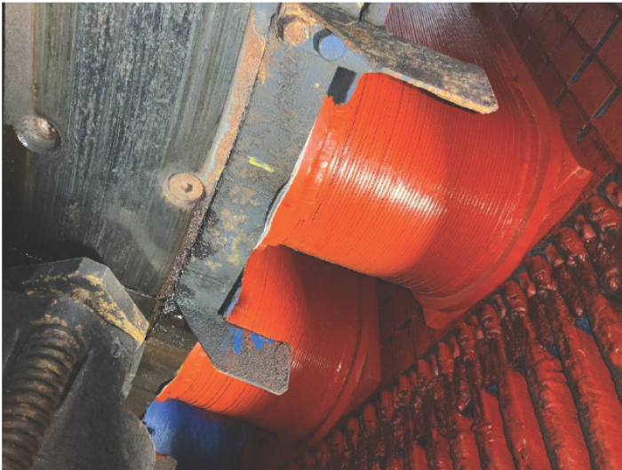
POLE 1 AND 44 WHICH WERE REFURBISHED IN 2023 AT DELSTAR ENERGY
