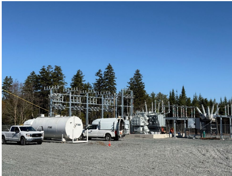
Figure 26: In Progress Construction of New Mount Uniacke Substation
