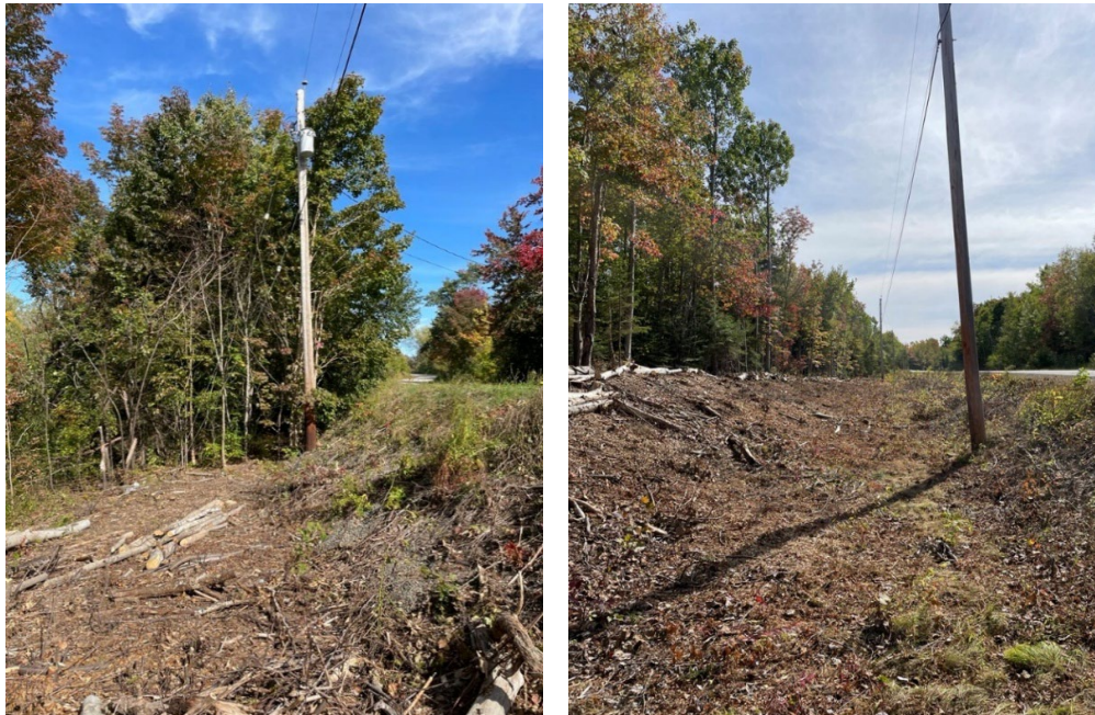
2 Figure 17: Egypt Rd, Between Trenton and Little Harbour- InProgress and Completed
