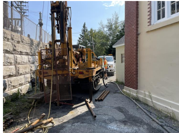
Photo 8: Drilling of borehole using CME-45 rig prior to monitoring well installation. Photo taken on September 11, 2024.
