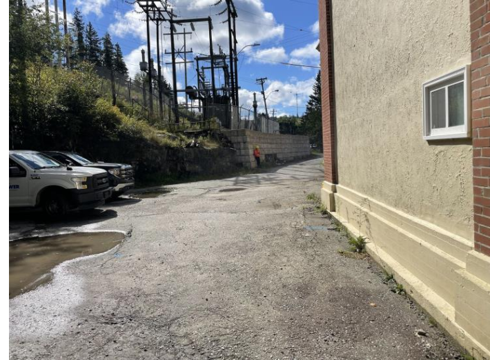
Photo 2: View of hydro-power plant and transformer substation on north side of the site, looking south. Photo taken on September 11, 2024.
