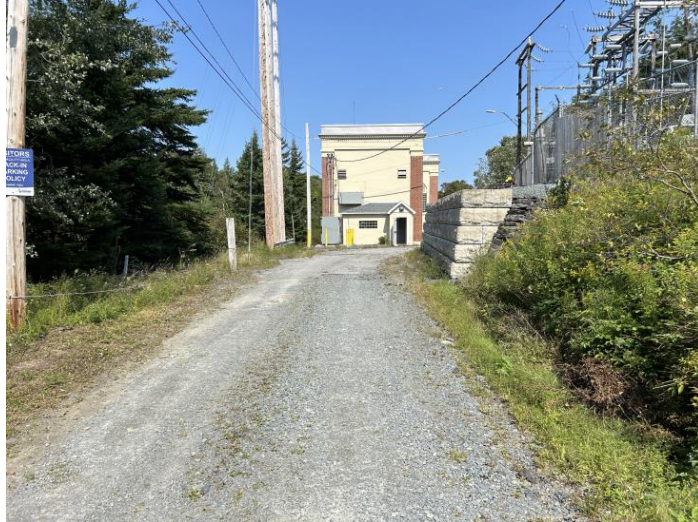
Photo 1: View of gravel driveway entry to the site and hydro-power plant building, looking north. Photo taken on September 5, 2024.
