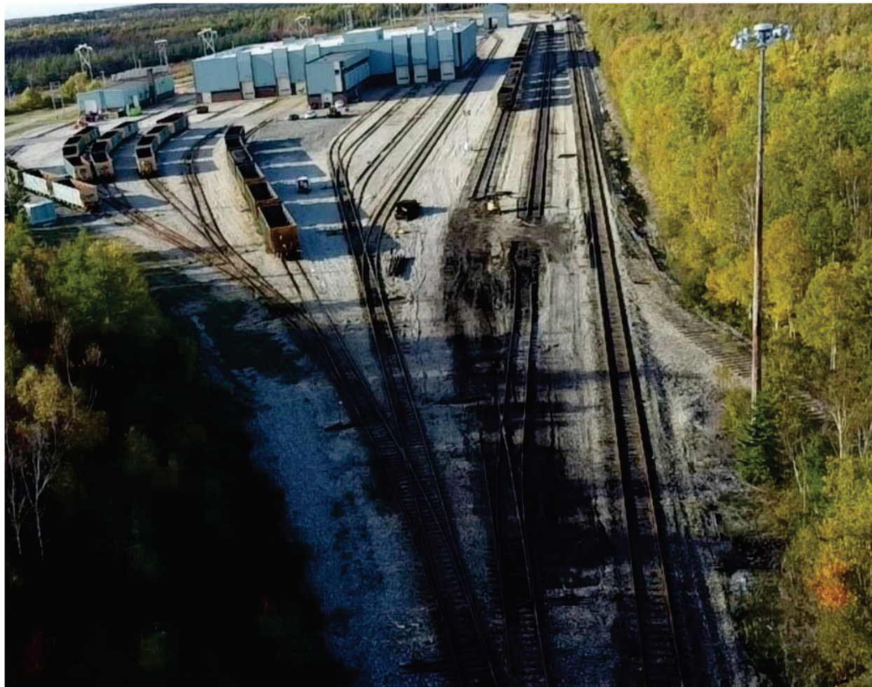
Figure V-10: Overhead photo of rail damage from derailment
