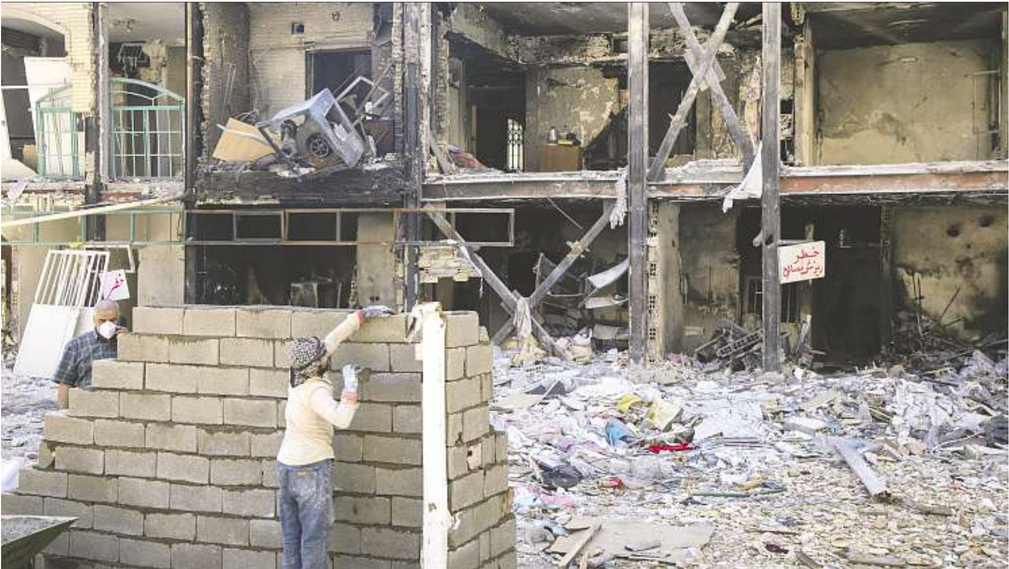
Workers build a wall at the site of a damaged residential building that, according to Iranian authorities, was hit by a strike on March 4 during the U.S.-Israeli military campaign, on April 14, 2026 in Tehran, Iran. On April 8 President Donald Trump announced a two-week ceasefire between the U.S. and Iran. Peace talks facilitated by Pakistan have since stalled, reportedly over Iran’s nuclear capabilities and control of the Strait of Hormuz. MAJID SAEEDI/GETTY IMAGES
