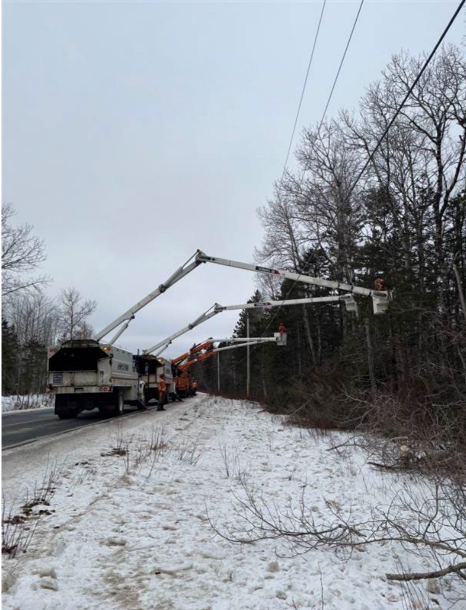
Figure 49 - Tree Trimming on 57W-402
