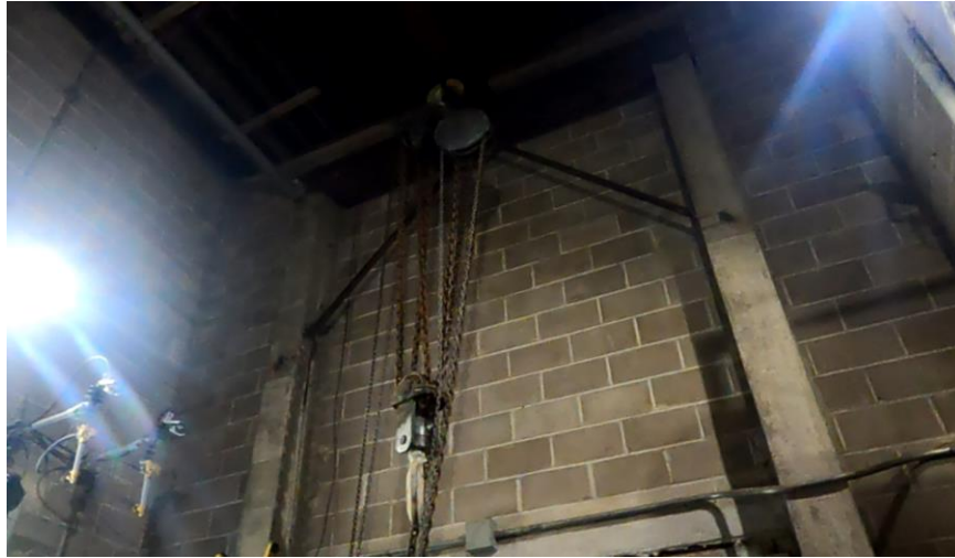
Figure 40: Columns and crane, east side, very good condition
