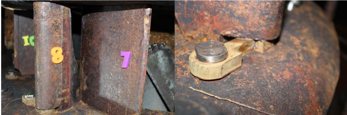
Figure 19: Wicket gate 8, half attached to the control link
