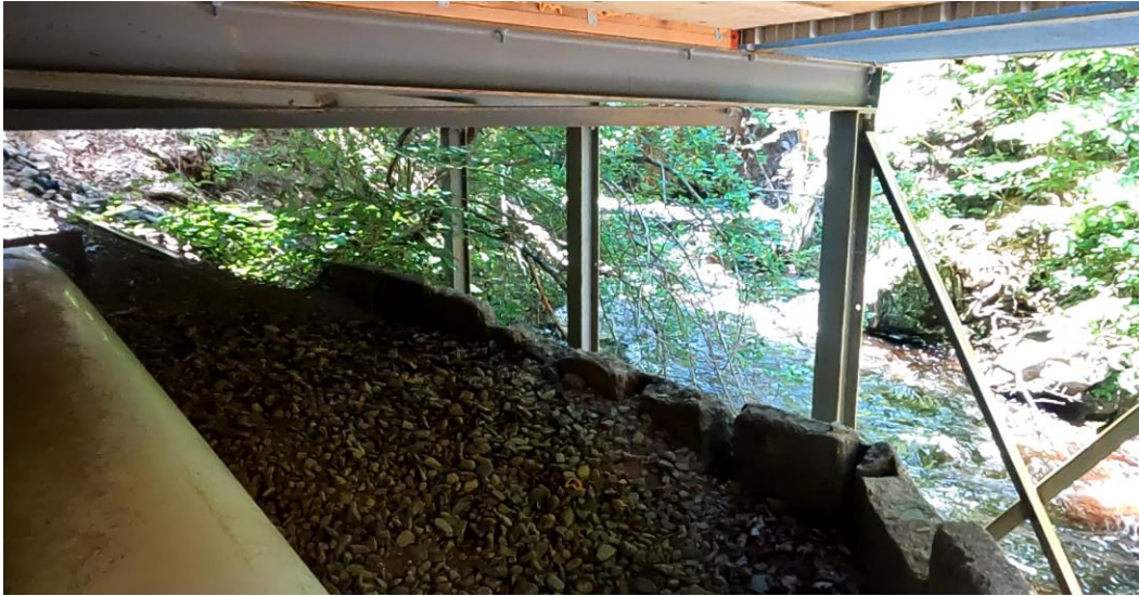
Figure 43: Gravel retainer wall
