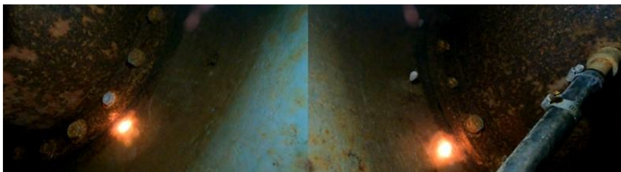
Figure 51: Bolts that attach the curb plate/scroll case to the draft tube, nothing out of normal
