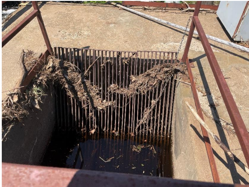
Figure 57: Trash rack
