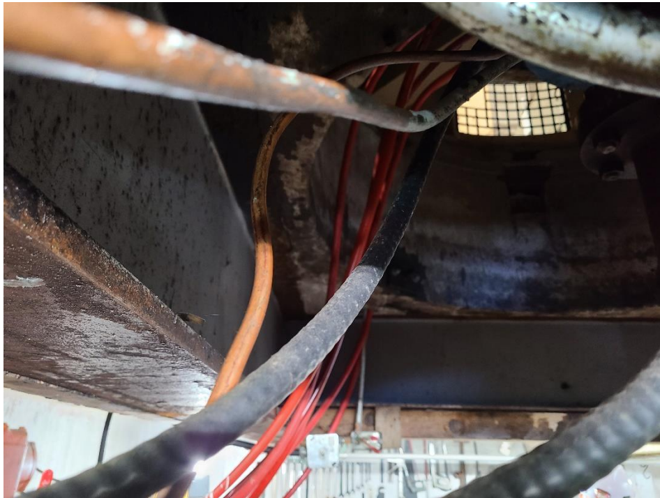
2. Steel beams around floor opening below generator.
