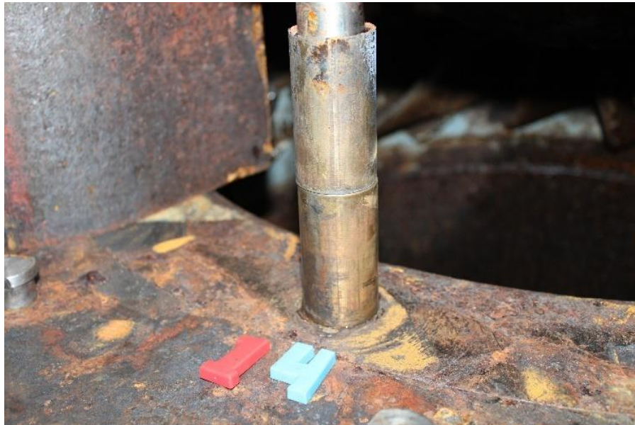
Figure 25: Wicket Gate 14 shaft, the only remain
