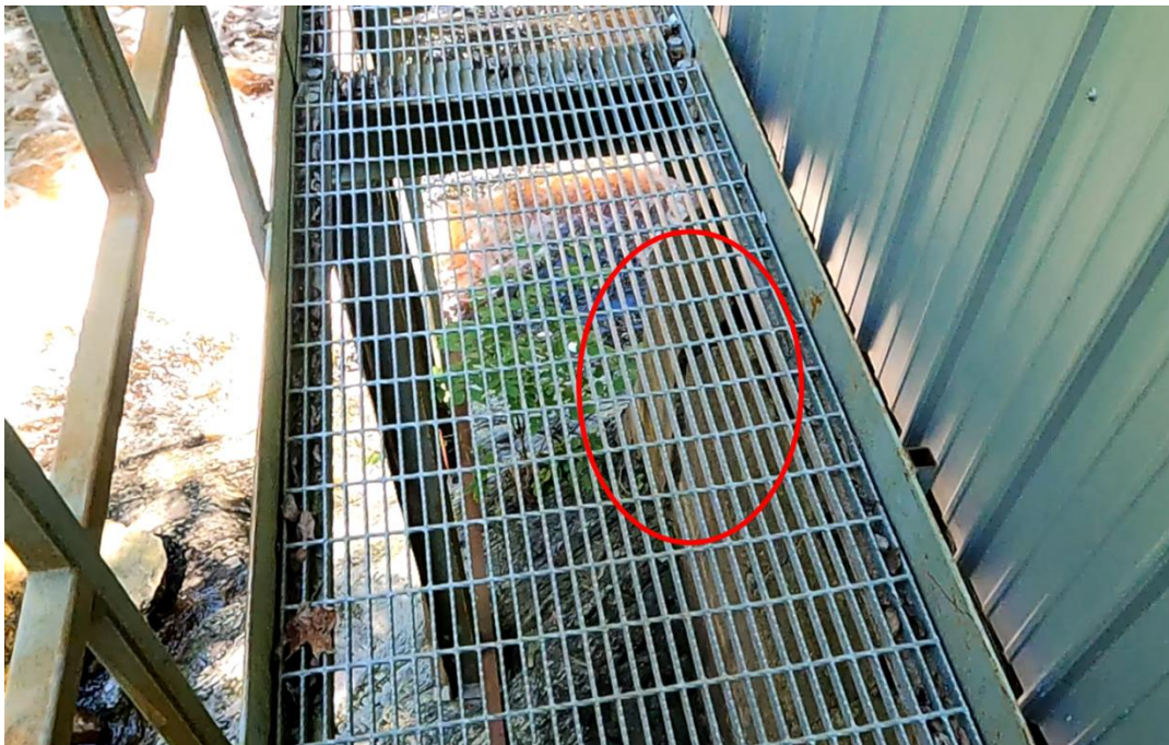
Figure 44: Crack on the retainer wall
