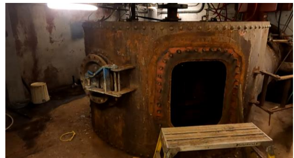
Figure 5: Scroll Case from the outside
