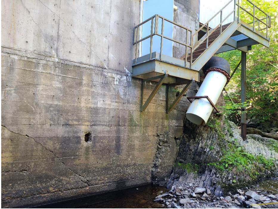
9. North face at Base Level.
