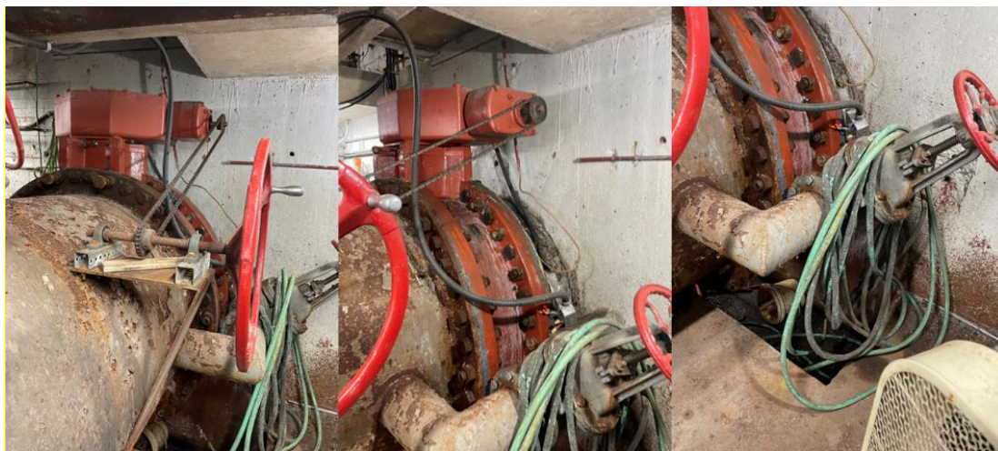
Figure 24: Intake valve.
