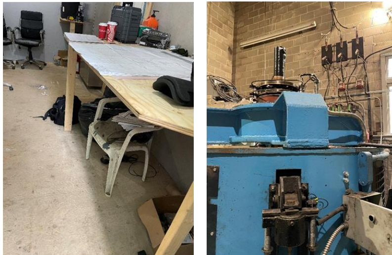
Figure 7: Powerhouse upper level.
