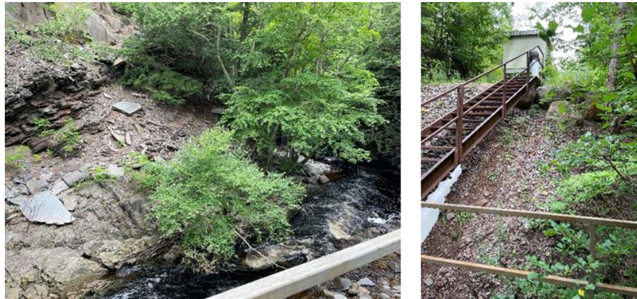
Figure 2: Slate slabs located around the powerhouse.
