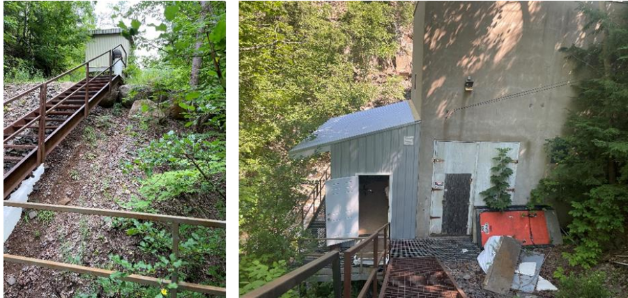
Figure 6: Draft Tube leading down from Surge Valve Building into the Powerhouse.
