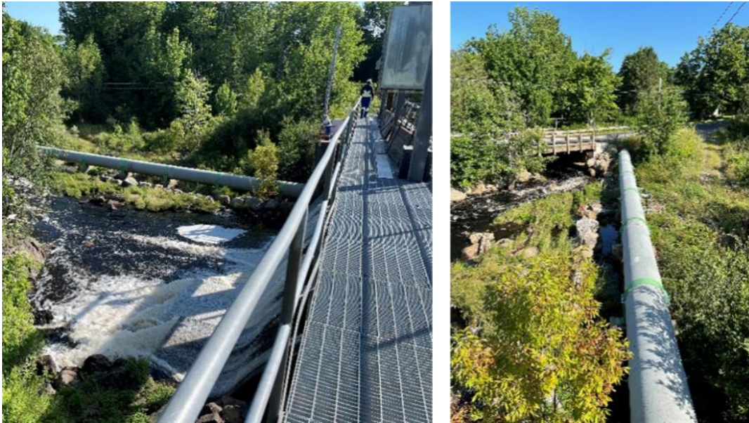
Figure 17: FRP section of draft tube looking downstream from dam.
