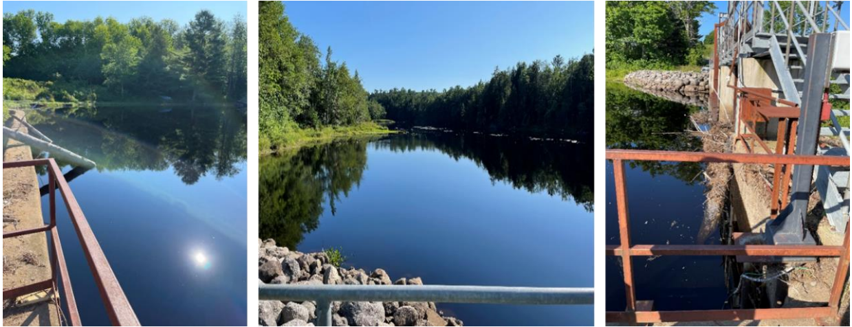
Figure 4: Head Pond views looking upstream from the dam.
