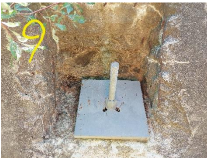
Photo 33 Post Tensioned Anchor #5-8 in Downstream Face of Right Dam Section
