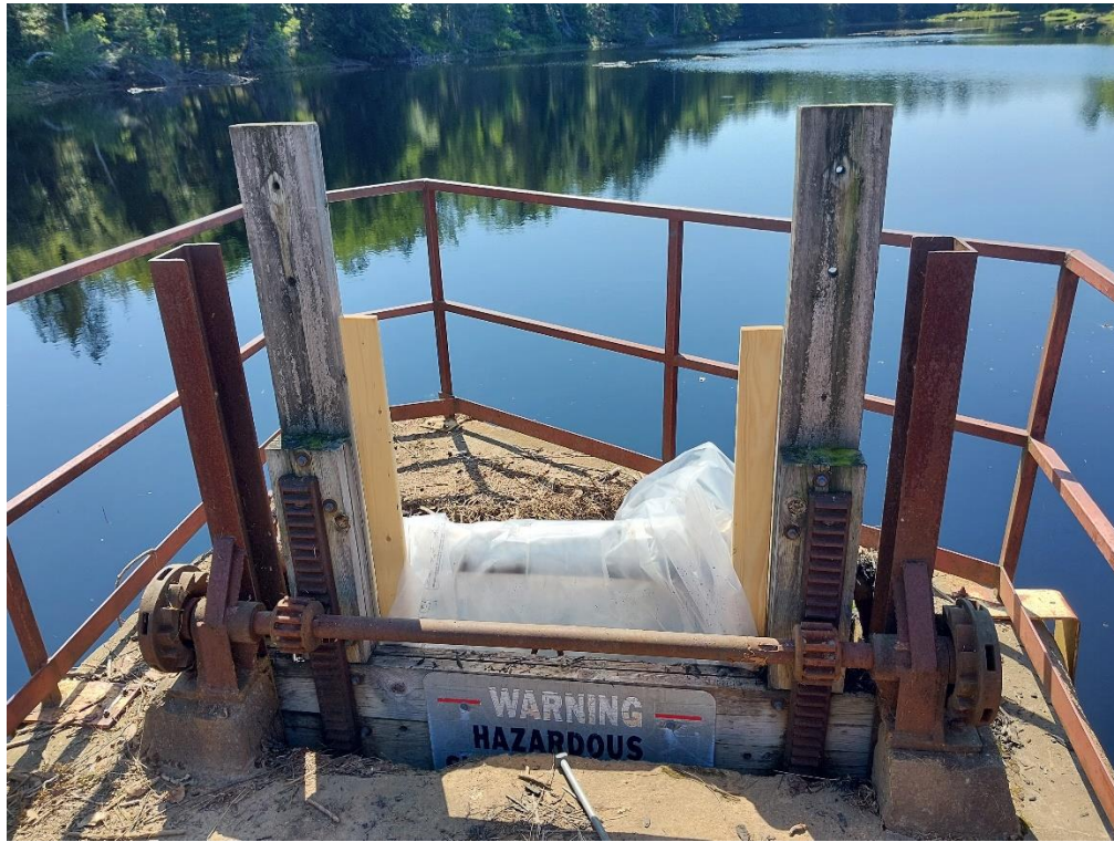
Photo 19 Plastic Seal in Front of Dewatered Intake Shaft
