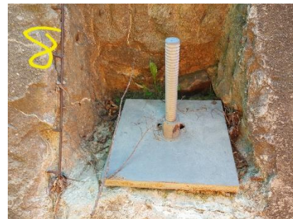
Photo 33 Post Tensioned Anchor #5-8 in Downstream Face of Right Dam Section
