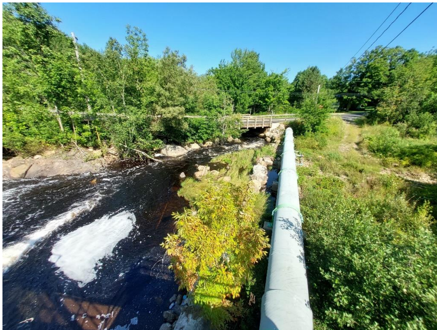
Photo 30 Penstock Alignment Looking Downstream from Intake
