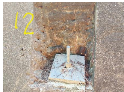
Photo 34 Post Tensioned Anchor #9-12 in Downstream Face of Right Dam Section
