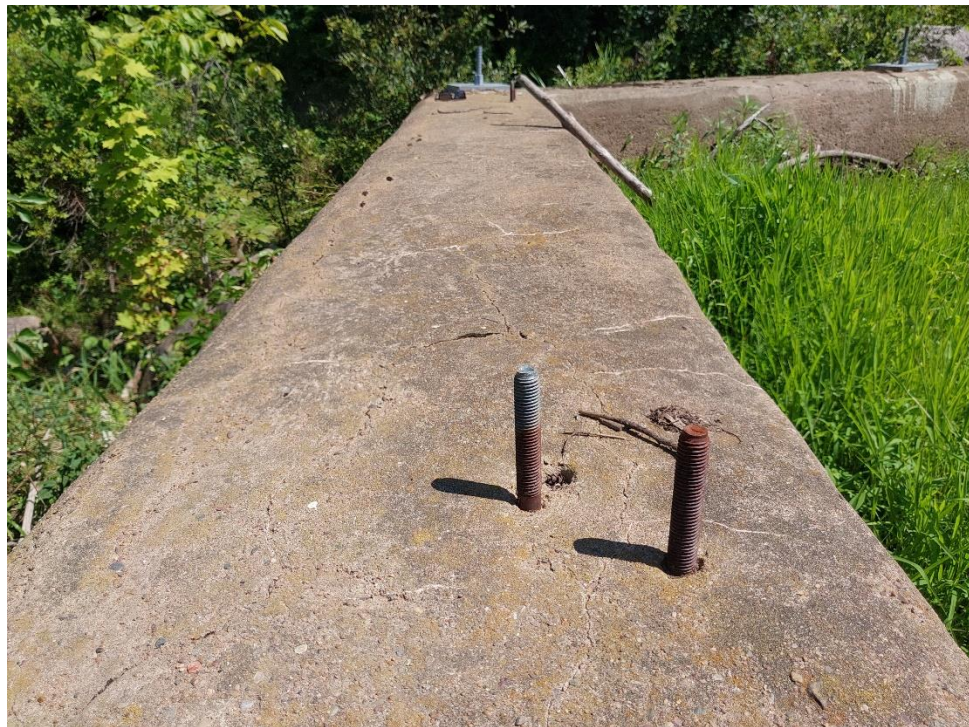
Photo 22 Bolts for Stoplog Gains On Right Dam Section
