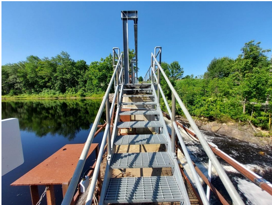
Photo 12 Stairs to Catwalk and hoist mechanisms
