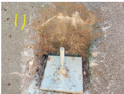
Photo 34 Post Tensioned Anchor #9-12 in Downstream Face of Right Dam Section
