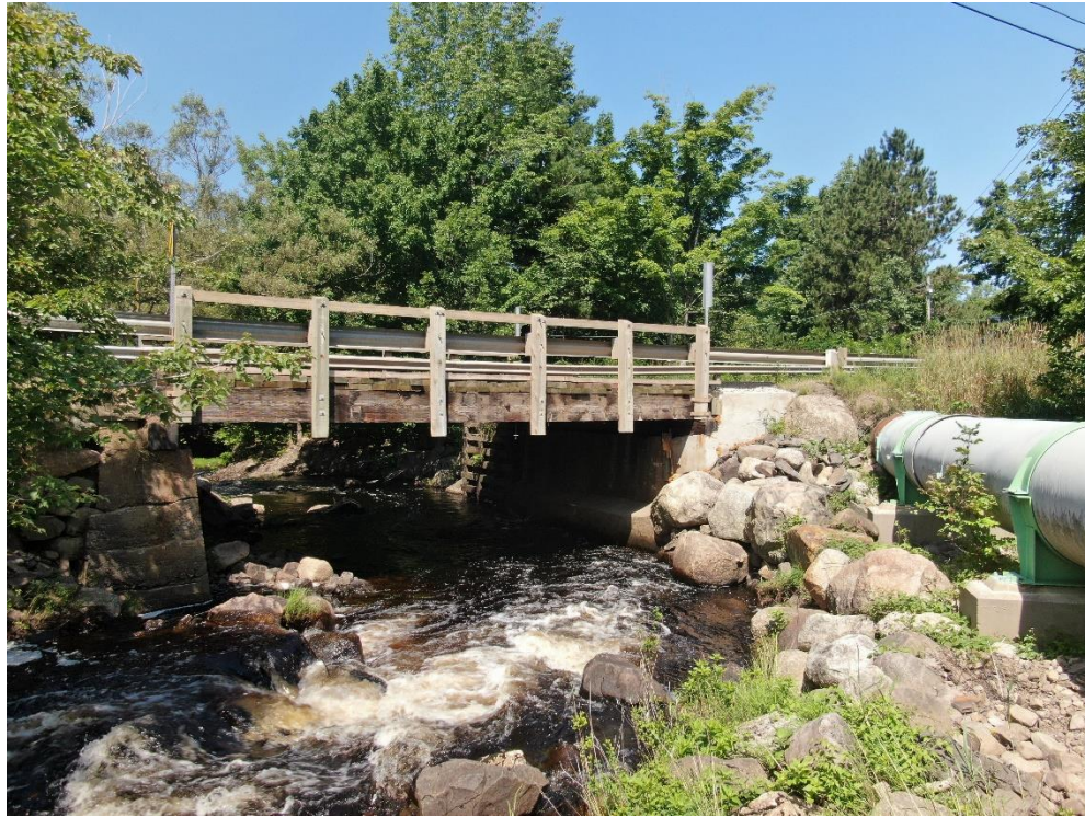
Photo 5 Downstream Bridge (Harmony Rd)
