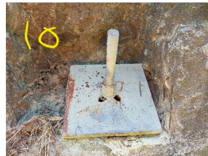
Photo 33 Post Tensioned Anchor #5-8 in Downstream Face of Right Dam Section
