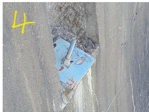
Photo 32 Post Tensioned Anchor #1-4 Starting at Exposed Part of Left Dam Section
