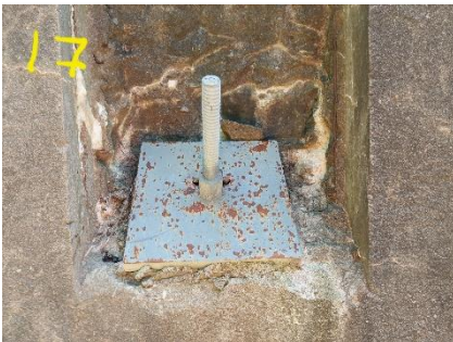
Photo 35 Post Tensioned Anchor #13-16 in Downstream Face of Right Dam Section
