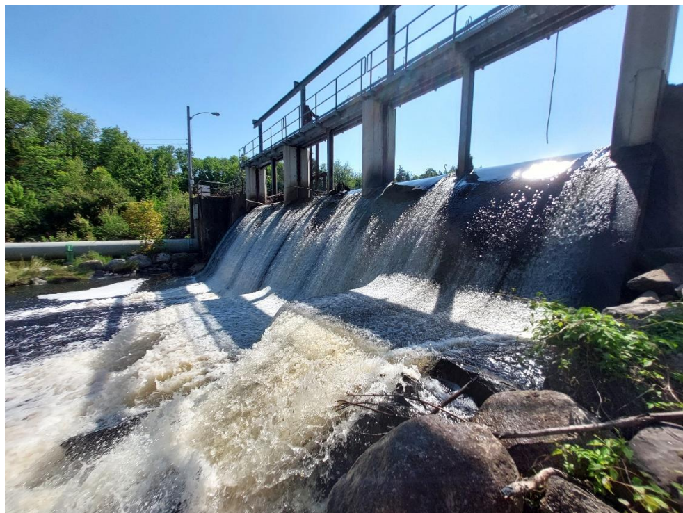
Photo 10 Spillway Looking from Left Side
