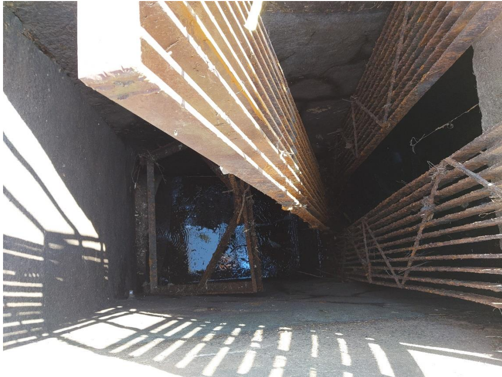
Photo 18 Looking into Intake Shaft Dewatered for Maintenance
