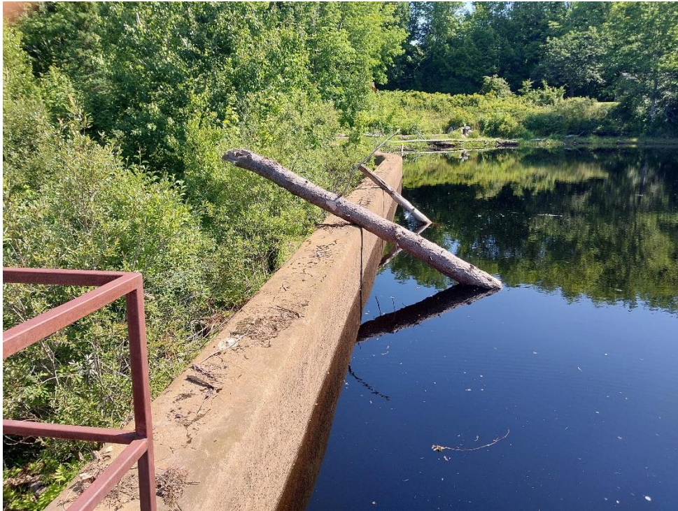
Photo 21 Right Dam Section Looking from Penstock Intake
