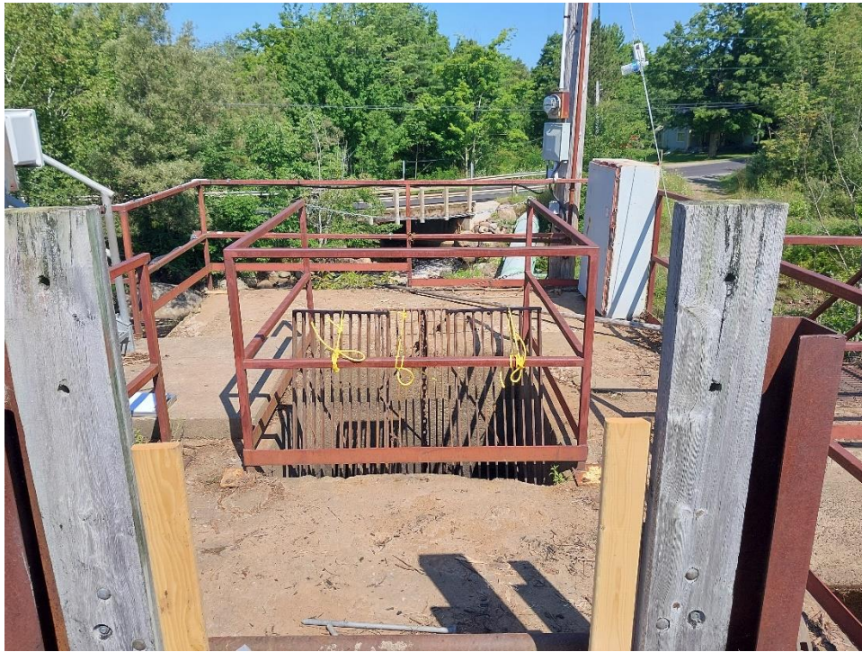
Photo 17 Dewatered Penstock Intake Shaft During Maintenance
