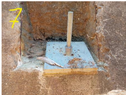
Photo 33 Post Tensioned Anchor #5-8 in Downstream Face of Right Dam Section
