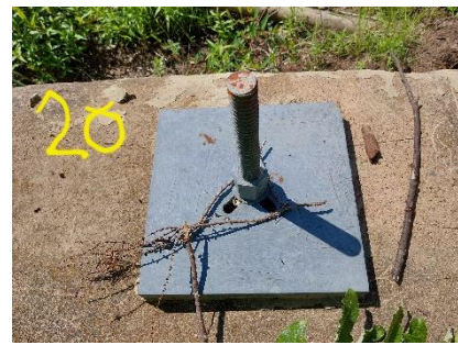
Photo 36 Post Tensioned Anchor #17-20 Ending at Top of Far Corner of Right Dam Section
