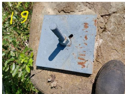
Photo 36 Post Tensioned Anchor #17-20 Ending at Top of Far Corner of Right Dam Section
