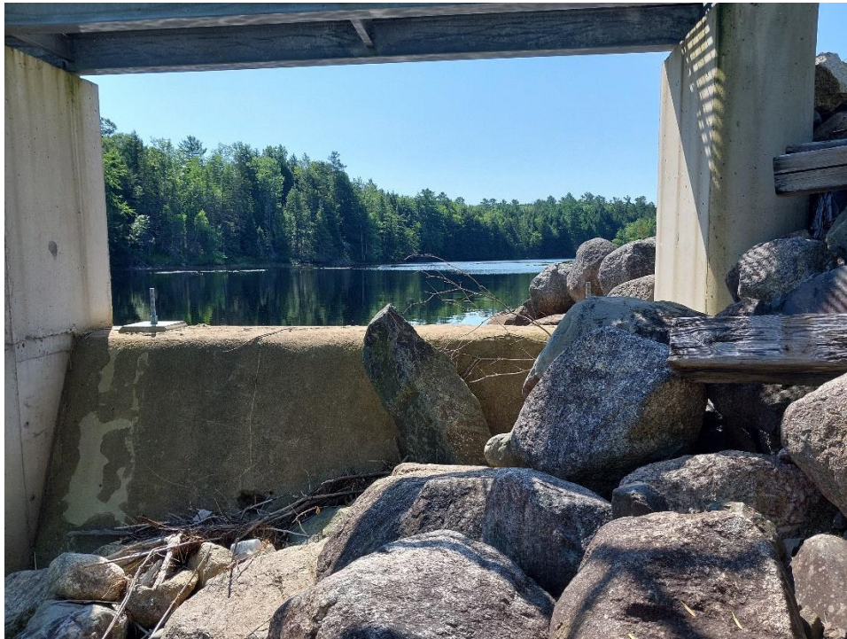
Photo 6 Exposed Portion of Left Dam Section
