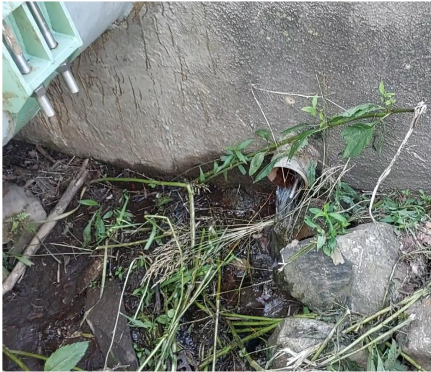
Photo 29 Drain Pipe Next To Penstock
