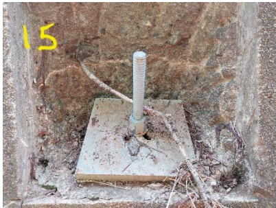
Photo 35 Post Tensioned Anchor #13-16 in Downstream Face of Right Dam Section
