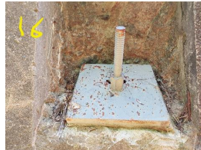
Photo 35 Post Tensioned Anchor #13-16 in Downstream Face of Right Dam Section
