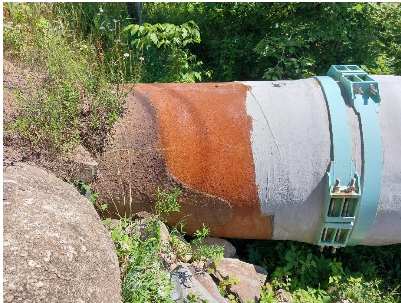
Photo 31 Penstock Passing Under Harmony Road Showing Rust
