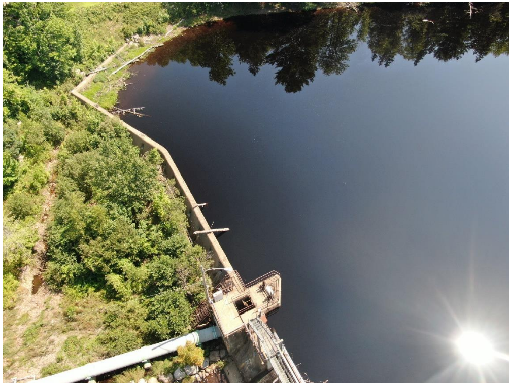
Photo 4 Right dam Section
