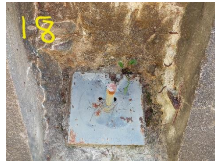
Photo 35 Post Tensioned Anchor #13-16 in Downstream Face of Right Dam Section
