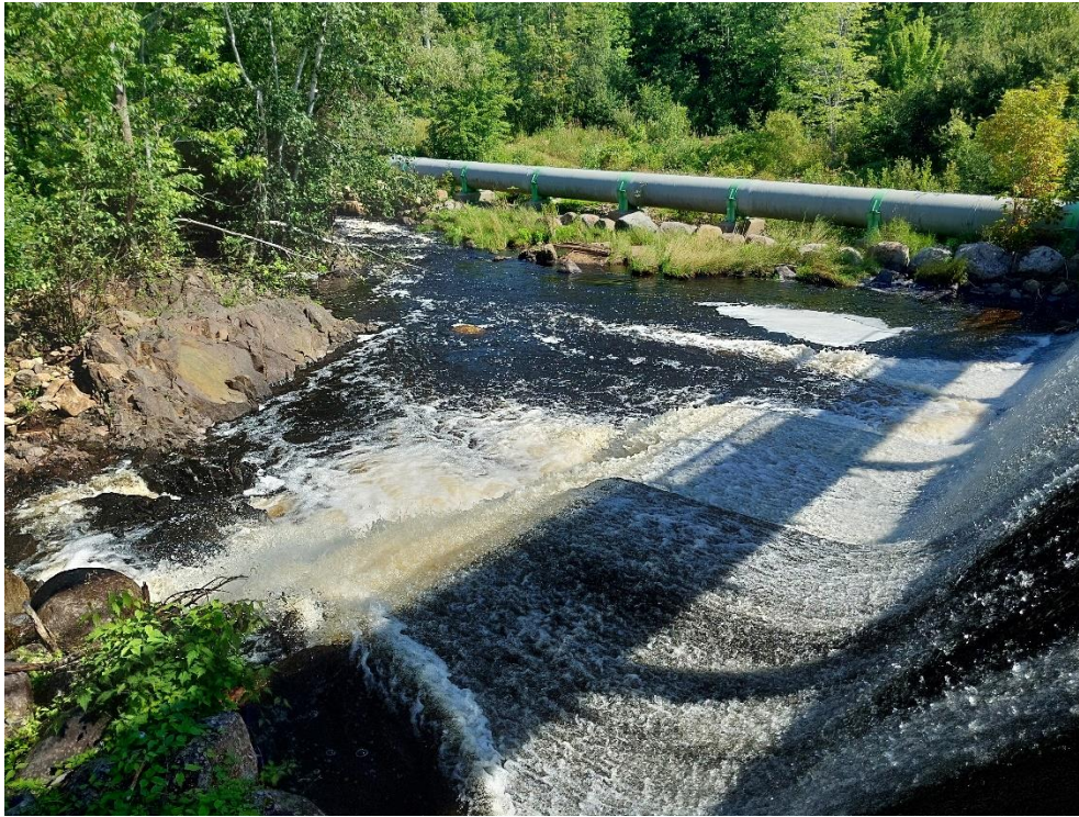
Photo 11 Tailwater of Spillway Looking from Left Side
