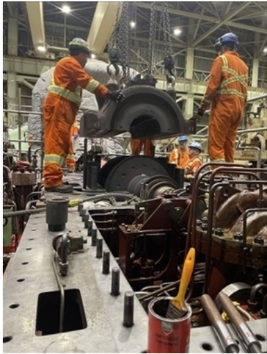
2.2.1.1 AF HP Inner Cylinder Lift
