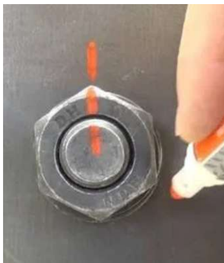
Figure 2 - Bolt Marking after torque
