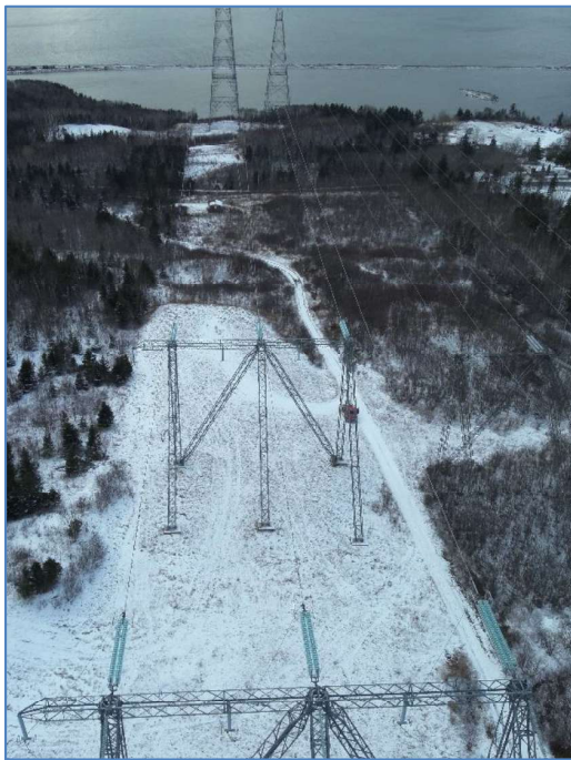
Figure 2 View along back span on Cape Breton Island from the drone. Structures supporting the new (left) and old (right) spans across the Canso Strait are shown in the far distance. Detail from Photo No. DJI_20240116015020_0011_Z.jpg
