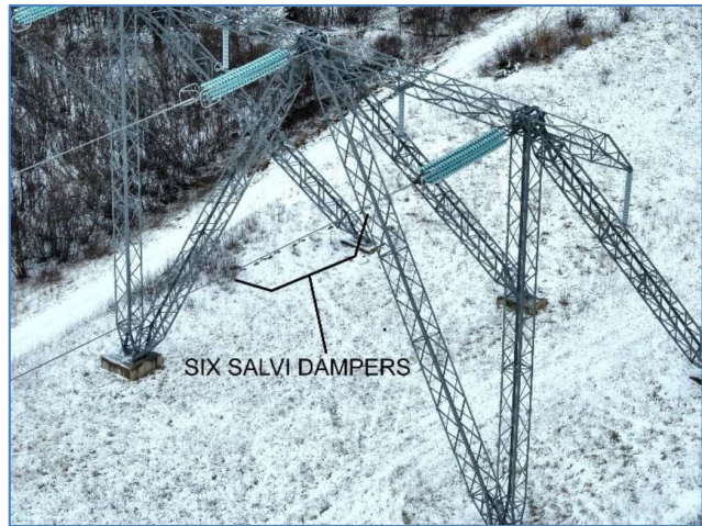
Figure 1 Dead end structure on Cape Breton Island from the drone. From photo No. DJI_20240116014927_0004_Z.jpg
