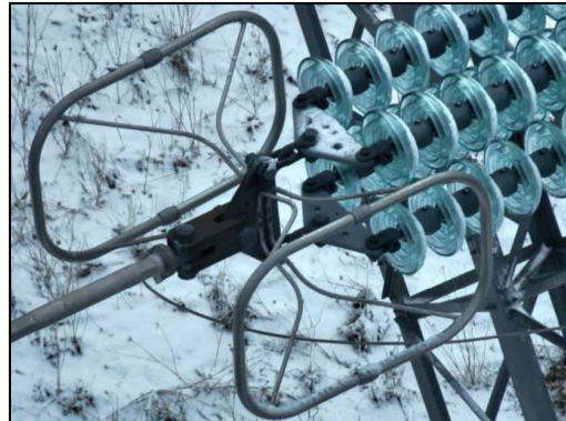
Figure 18 High voltage end of insulators on the dead-end structure on the back span on the Nova Scotia Mainland Detail from Photo No. DJI_20240116031655_0029_Z.jpg
