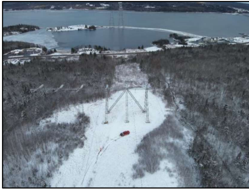
Figure 15 View of the back span looking north towards the suspension structures on the Nova Scotia Mainland. Detail from Photo No. DJI_20240116031218_0001_w.jpg
