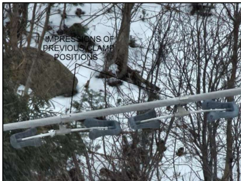
Figure 19 Conductor impressions where previous Salvi damper clamps were located, or clamp slippage had occurred on the back span on the Nova Scotia Mainland. Detail from Photo No. DJI_20240118000131_0025_Z.jpg
