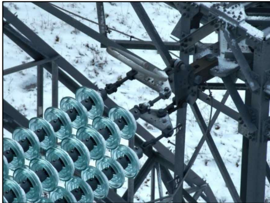
Figure 17 Ground end of insulators on the dead-end structure on the back span on the Nova Scotia Mainland. Detail from Photo No. DJI_20240116031651_0028_Z.jpg
