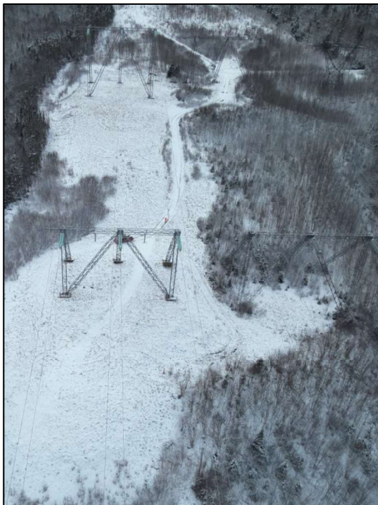
Figure 16 View looking south showing dead end structures on the back span on the Nova Scotia Mainland. Detail from Photo No. DJI_20240116031338_0010_w.jpg
