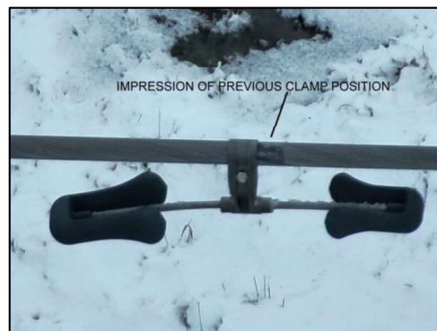
Figure 20 Conductor impressions where Salvi damper clamps were located or clamp slippage had occurred on the back span on the Nova Scotia Mainland Detail from Photo No. DJI_20240116031756_0035_Z.jpg
