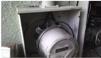
Bypass conductors installed
