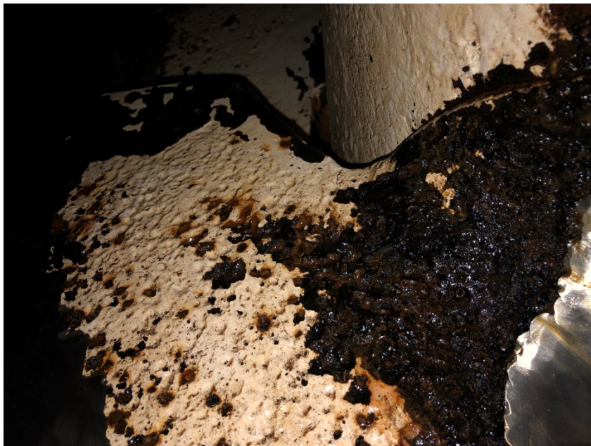
Runner blade - Very poor condition.
