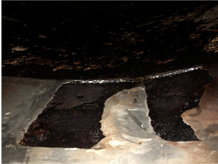
Bottom Right hand corner of draft tube door is eroded from old vacuum pipe. Inspection door is also cracked up the center.
