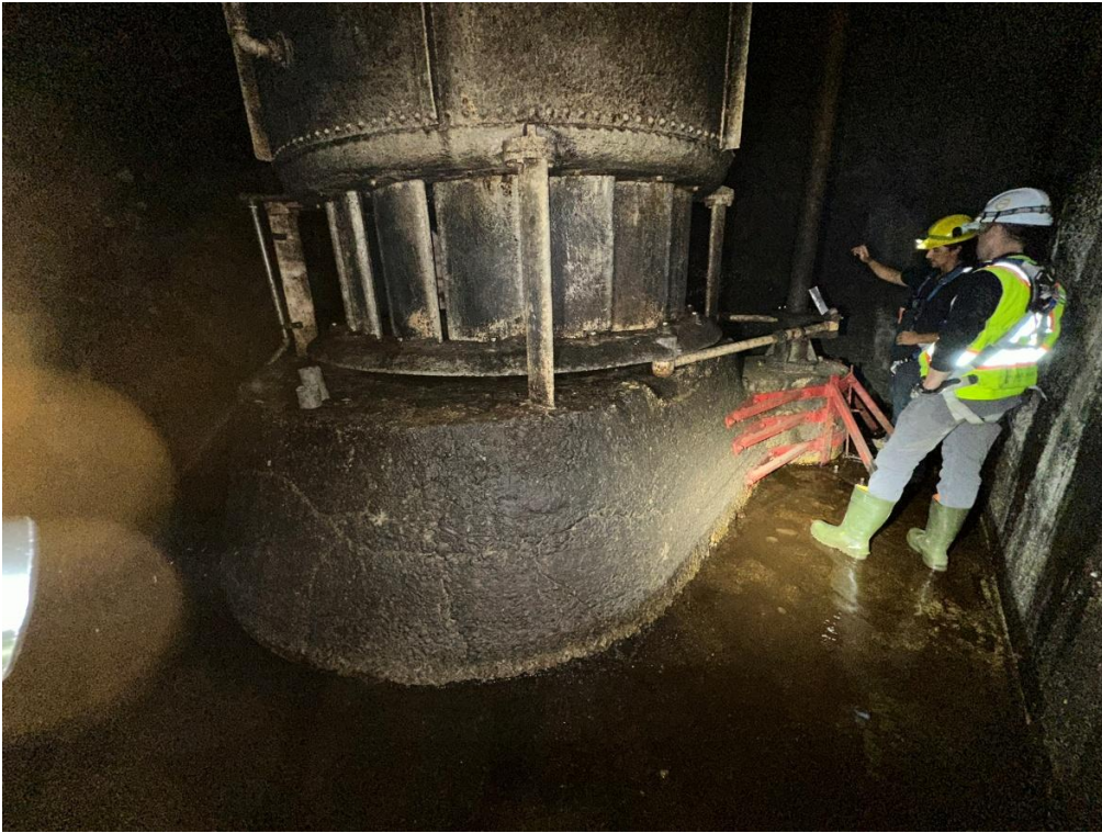
Figure 3: Main concrete pedestal supporting draft tube; Concrete block supporting quadrant shaft on right
