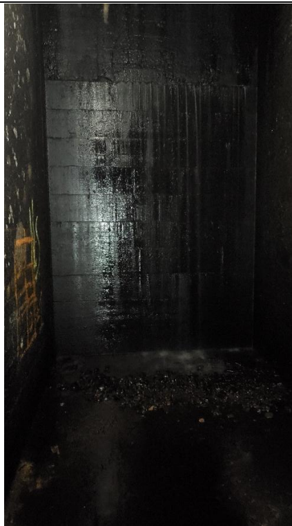
Figure 10: Water leakage at stop logs
