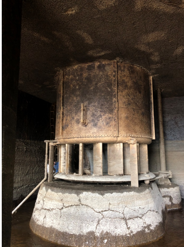
Repositioned and welded to correct misalignment
