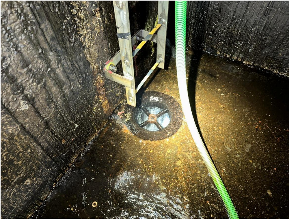
Figure 9: Drain located at corner with entrance ladder
