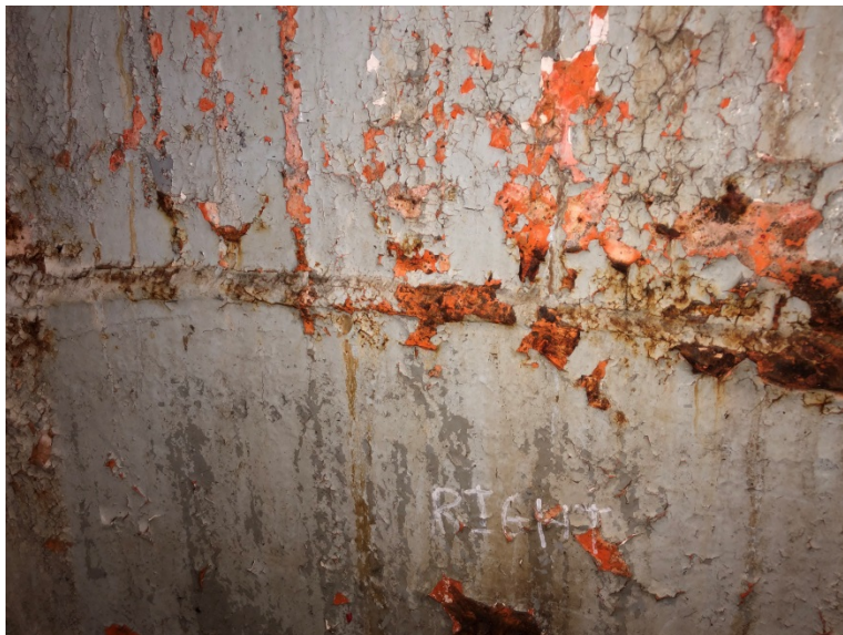
Repositioned and welded to correct misalignment
