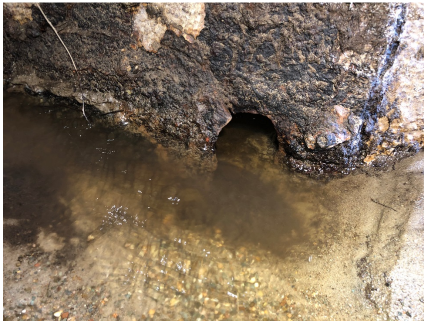
Bottom Right hand corner of draft tube door is eroded from old vacuum pipe. Inspection door is also cracked up the center.
