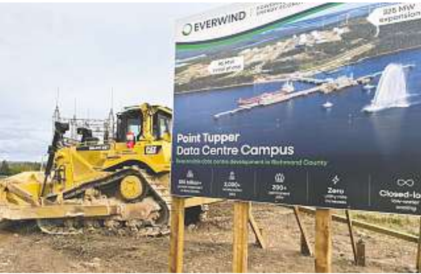
Construction equipment sits next to a sign at the future site of a green hydrogen plant and data centre in Point Tupper. PHOTOS: AARON BESWICK/POSTMEDIA NEWS
